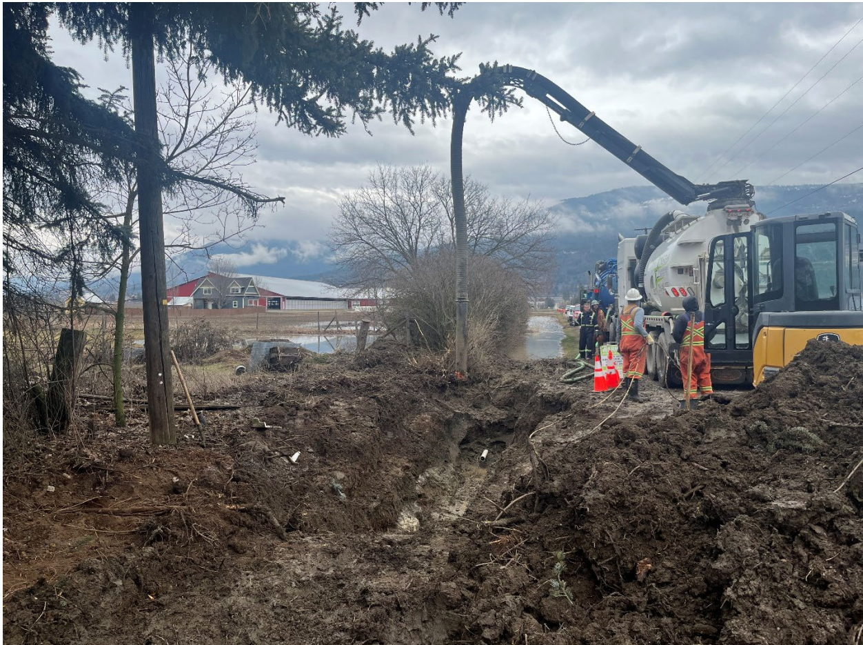
Photo Credit: Larkin Cross Road Main Repair
