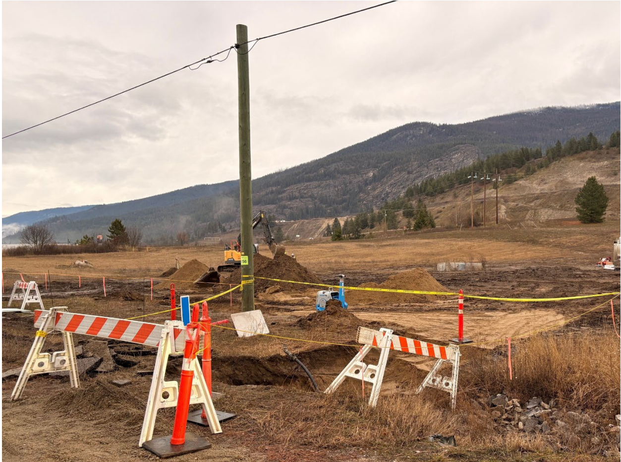
Photo Credit: Well 6 Construction Begin
